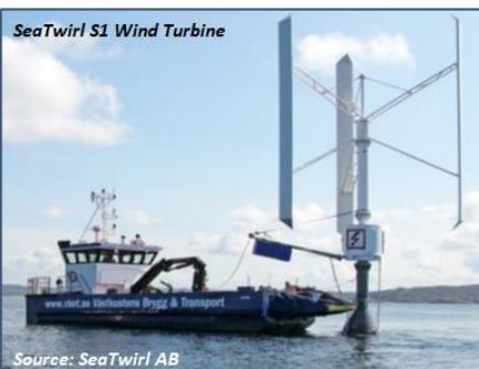
Thanks to the floating sub-sea structure of the wind turbine, the bearings inside the generator housing do not need to carry the weight of the turbine. This is unique to *SeaTwirl* and means that the bearings are subjected to less loads than in other wind turbines. *SeaTwirl's* wind turbines have a lower centre of gravity and a more stable design than horizontal-axis wind turbines, because the generator and all parts
